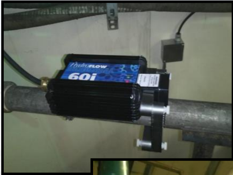
Installed HydroFLOW equipment
