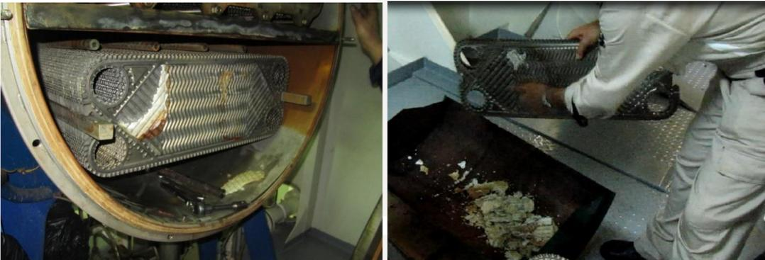
**Figure 9.** Some plates had limescale on them, but it was easily removed by hand.
