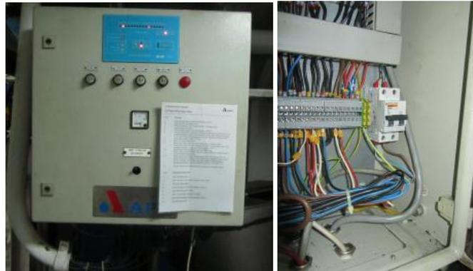
**Figure 7.** FWG main power cabinet and cable connection.
