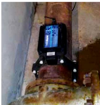
The HydroFlow system allowed pool staff to reduce the amount of chemicals used in the pool.
