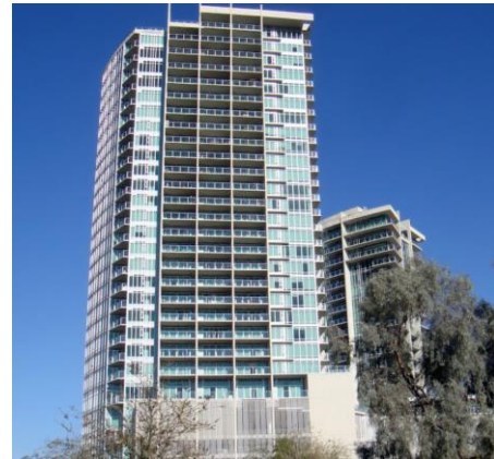
West Sixth Residential Towers - Tempe, AZ
